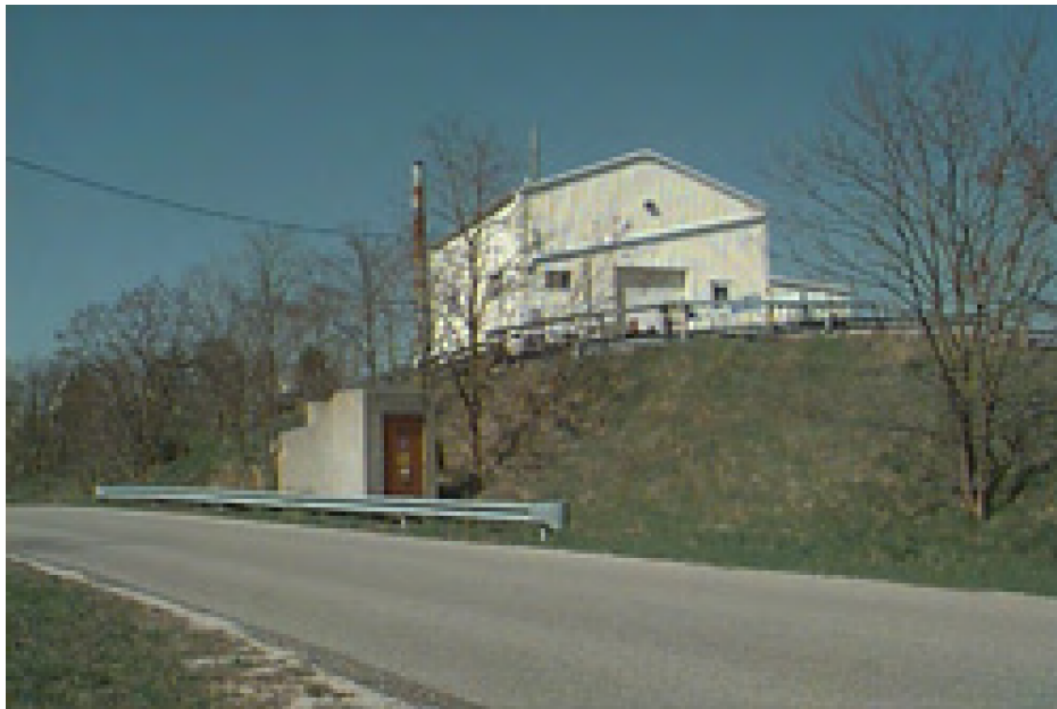
Figure 2. The BLIP facility.
