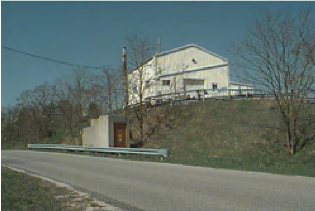
Figure 2. The BLIP facility.
