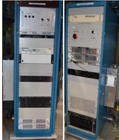
Fig.7: Two power supplies (one for inner and one for outer) – each power supply has its own set of dump resistors for fast energy extraction.
