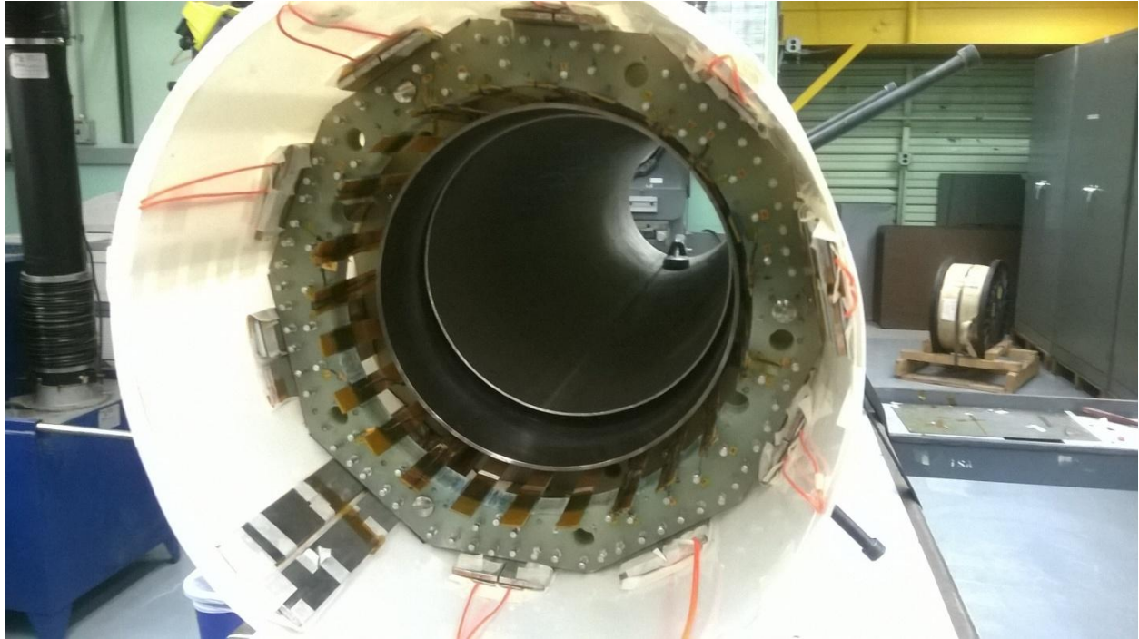
Figure 10: A view of leads, etc. from one side of outer coil during the construction.
