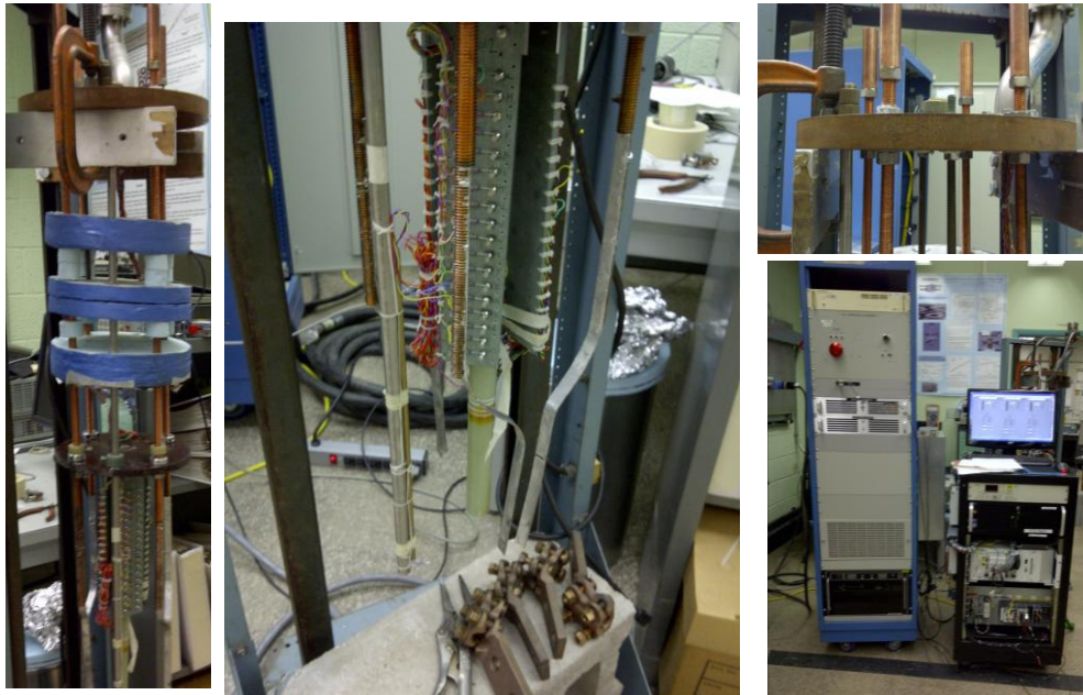
Fig. 10: Views of recently upgraded top-hat and power supply, etc. to test coils to \sim 1000 A.
