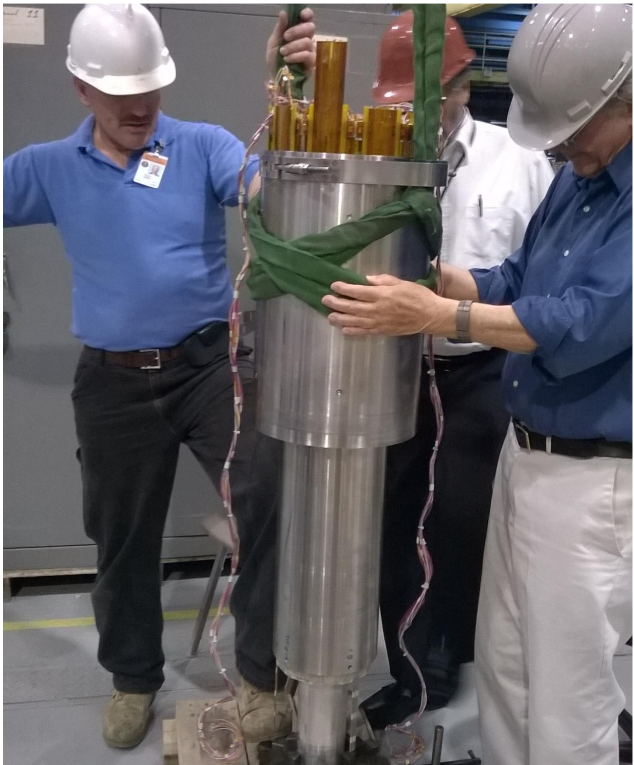
Figure 2: Outer coil with support structure being inserted over the inner coil with support structure.
