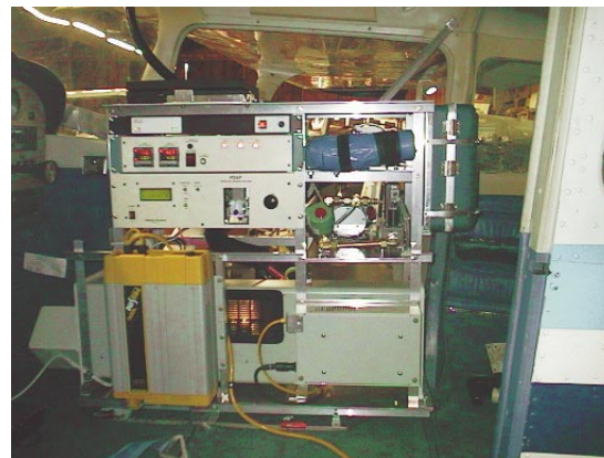
Port view of rack
